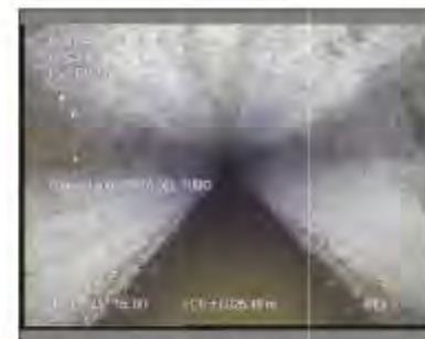
Foto: 21_1_5_18022021_160300_A.JPG 25,4m, Comentario
